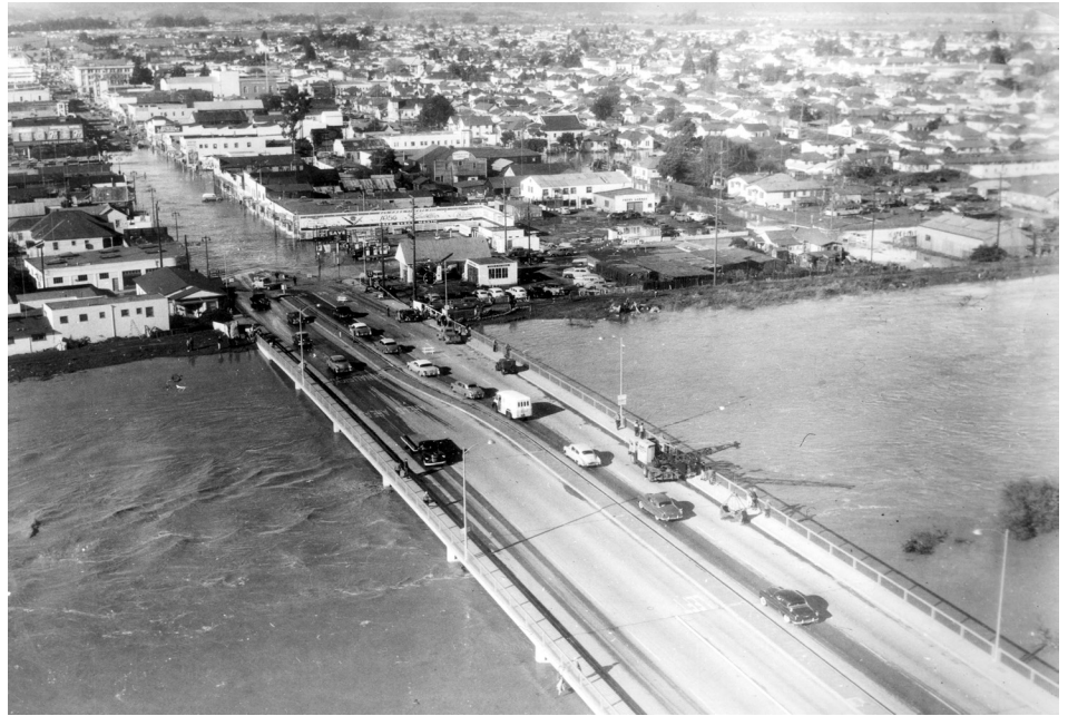
Granite Construction's crane on the Main Street bridge moving debris to the other side of the bridge to allow the water to flow during the flood of December 23, 1955.
