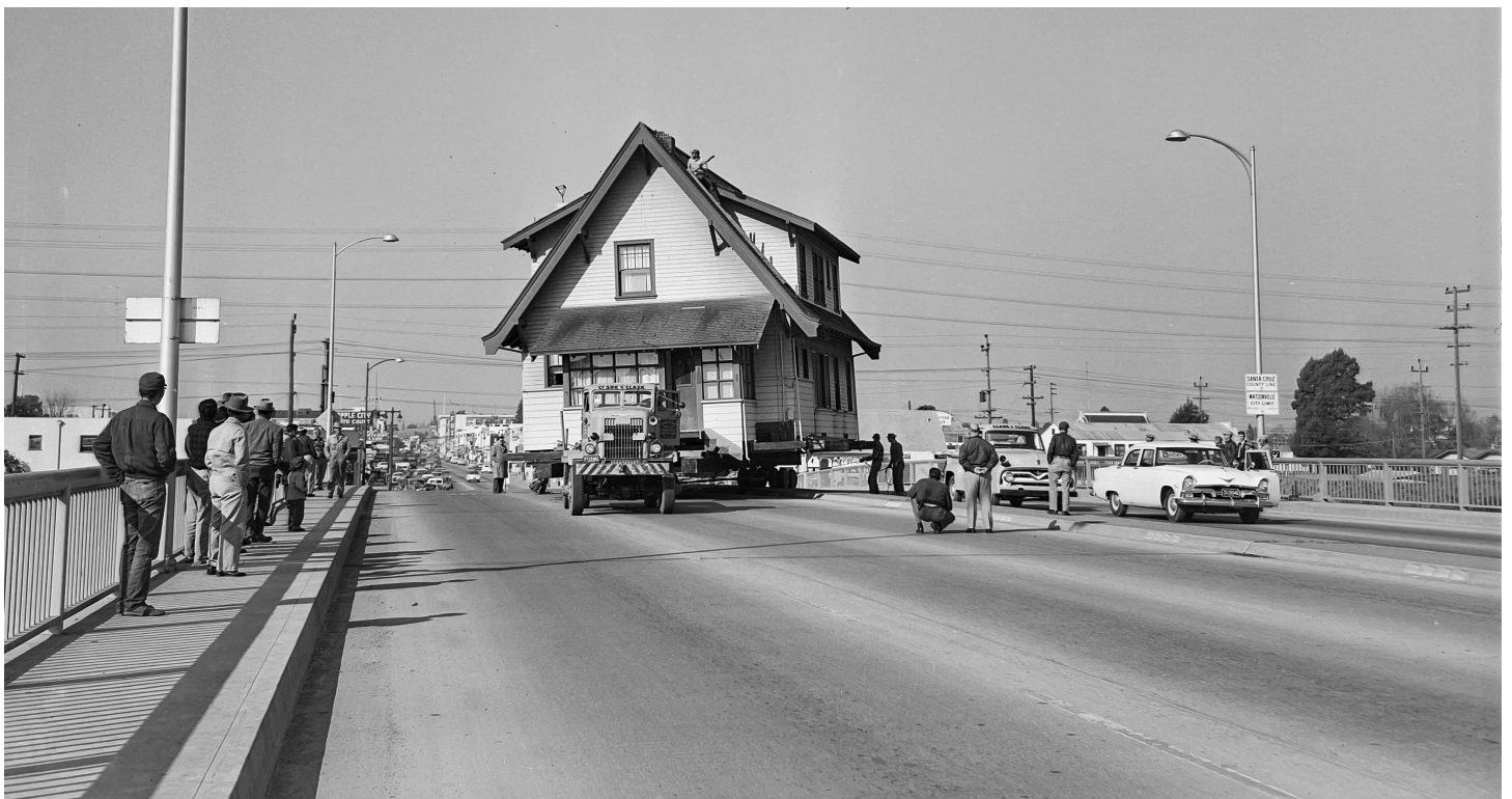
A house formerly on East Lake Avenue was moved to Pajaro in 1955, to serve as a parish house for the Church of the Assumption.
