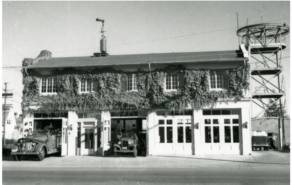
The fire station (now a museum) was built in 1924. After the great fire of 1927, two new bays were added to the building and a 60-foot steel tower was erected on which firemen could practice.
